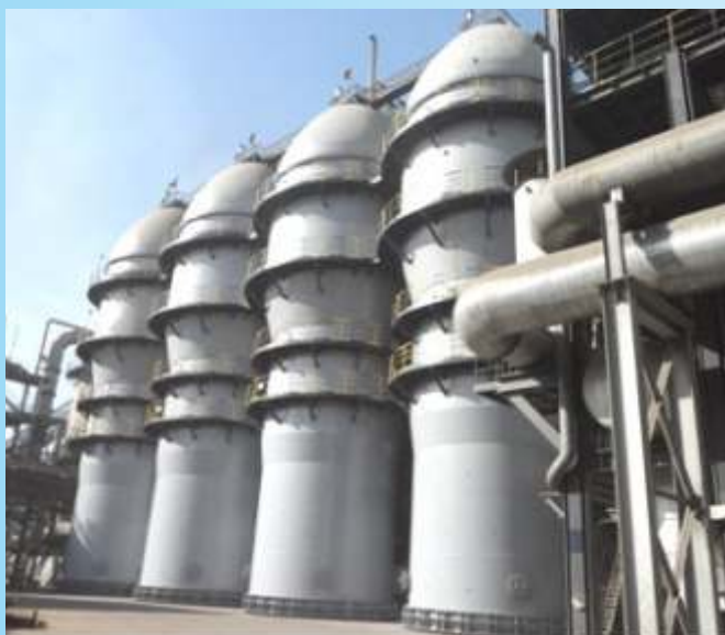
Yuxing top fired stove with a catenary dome achieved monthly mean HBT of 1314.7 °C
