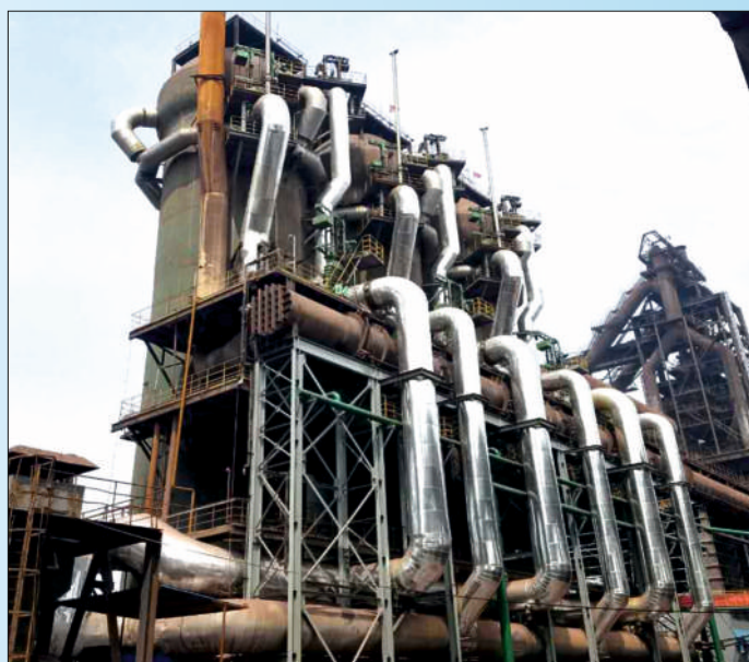
Internal combustion chamber stoves for 1497m 3 BF at JianLong Steel converted into Yuxing top fired with a catenary dome
