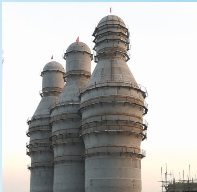
3x3580m 3 BF's configured with Yuxing 4-section top fired stoves
